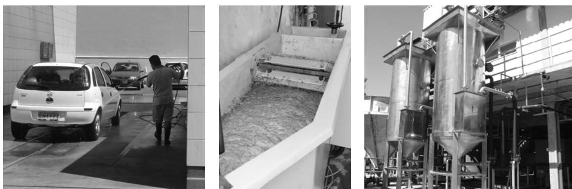
Figure 11. FF applied for the water treatment and reuse from cars, buses and airplanes washing units (Porto Alegre/Brazil).
